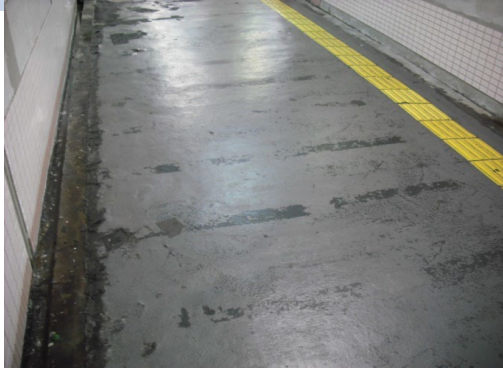
First day 0 : 30 start to clean up
