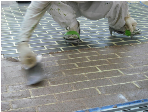
Surface coat by iron leveling
