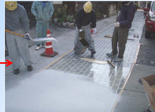
11:00 Apply MMA binder on the floor and distribute aggregate
